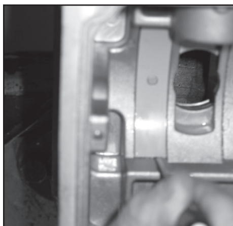
Removal of cradle bearings
